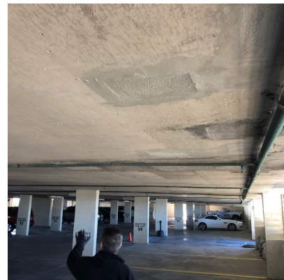
Repaired garage ceiling
