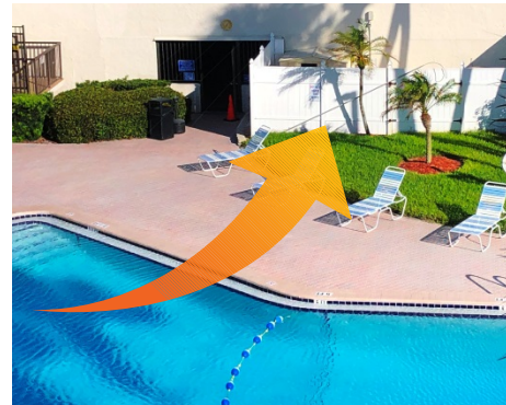
Heaters, filters & pumps are behind the white fence
