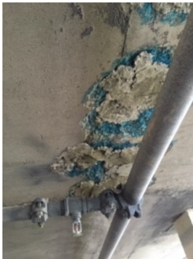
Rebar corrosion
